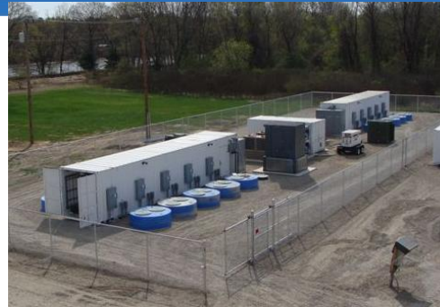
2 x 1MW / 15 min Flywheels in NE-ISO
