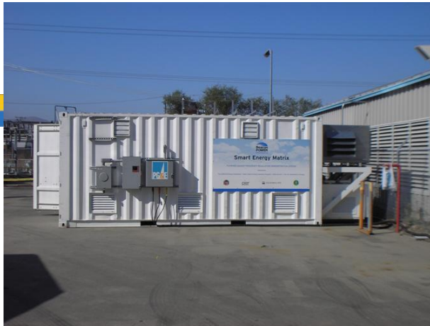
100kW/15 min Flywheel system Demos CEC / DOE and NYSERDA / DOE
